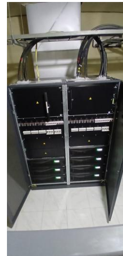
CumulusPower™ open frame — 7 independent modules
